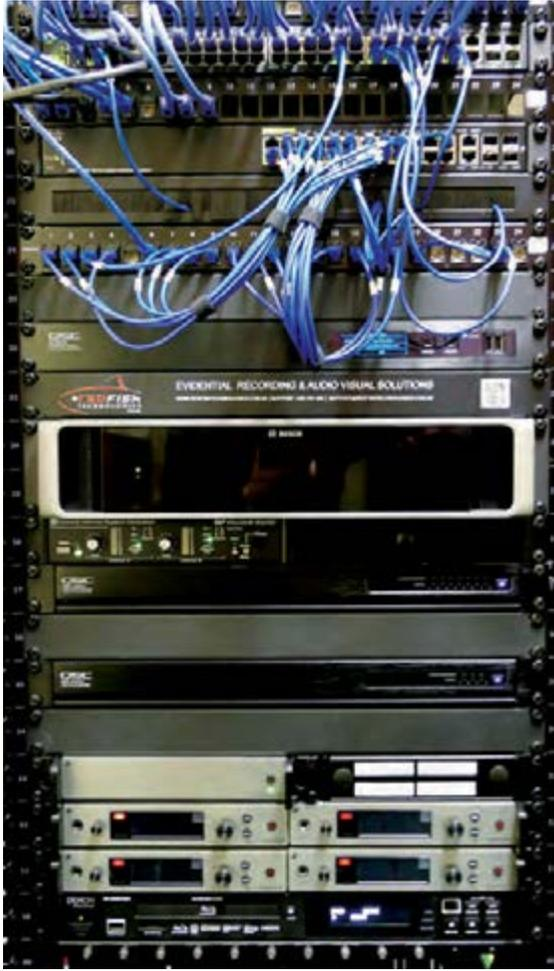
**Cat-6a cabling connects to a Cisco SG350 network switch in the rear room equipment rack**
